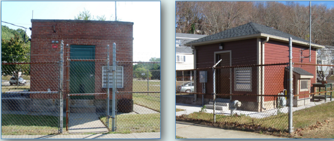
Mill Rock Pump Station before and after rehabilitation
