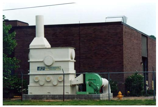
Figure 9-4. Photograph of a Chemical Scrubber
