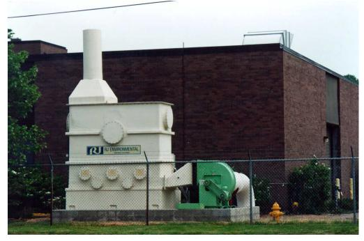
Figure 9-4. Photograph of a Chemical Scrubber
