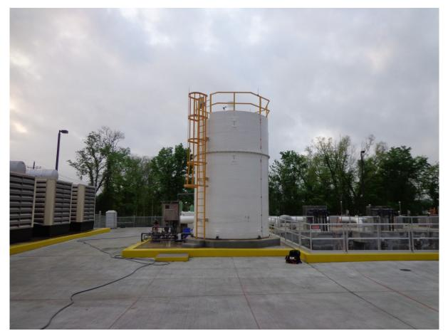
Figure 9-2. Photograph of a Biotower System
