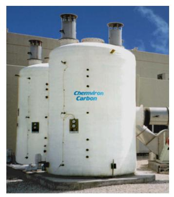
Figure 9-4. Photograph of a Dual Bed Carbon Scrubber
