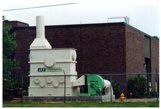
Figure 9-5. Photograph of a Chemical Scrubber
