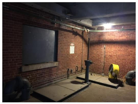
Figure 7-1. Building Access Hatches and Vent Pipes
