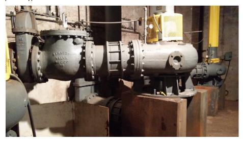
Figure 2-2. Suction and Discharge arrangement for Pump 2
