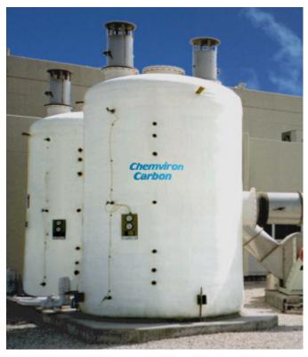
Figure 9-4. Photograph of a Dual Bed Carbon Scrubber
