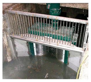
Figure 2-4. Typical Grinder Installation
