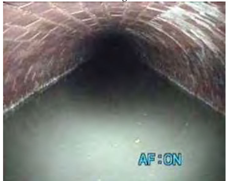
View of flow through effluent line
