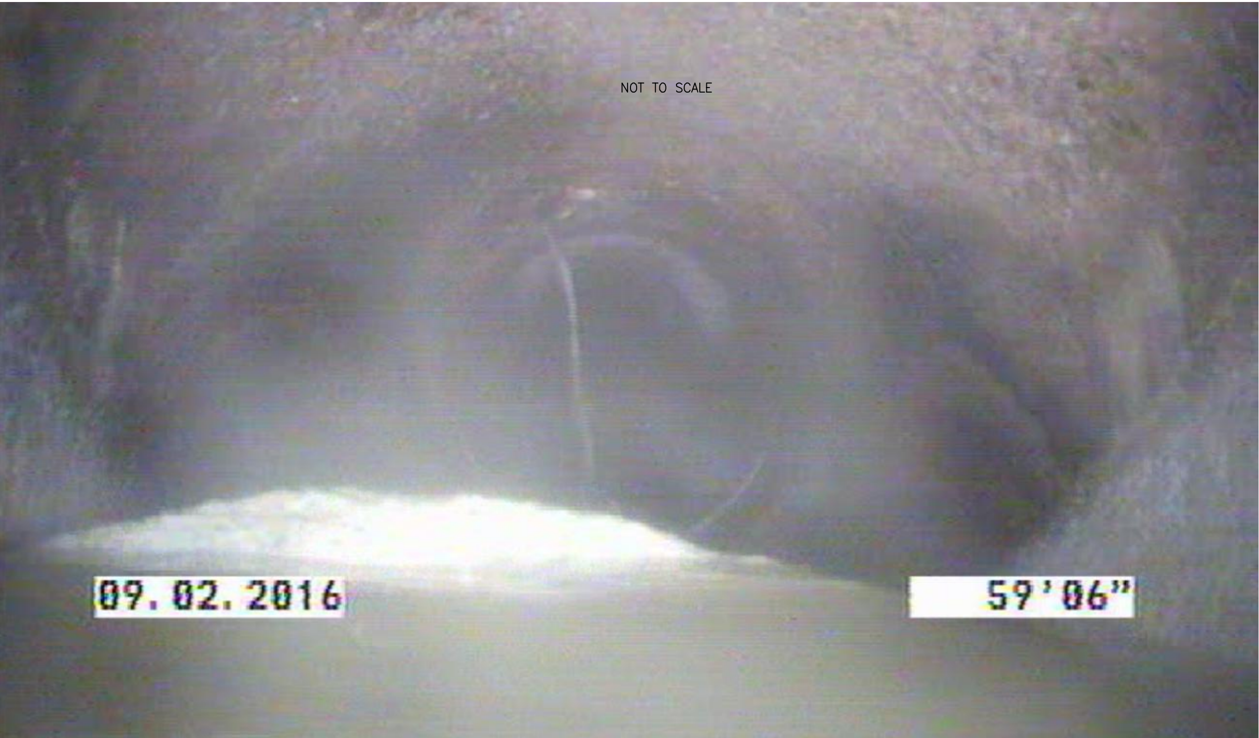
DEBRIS BETWEEN MH-NQL01M0152 & MH-NQL01M0153
