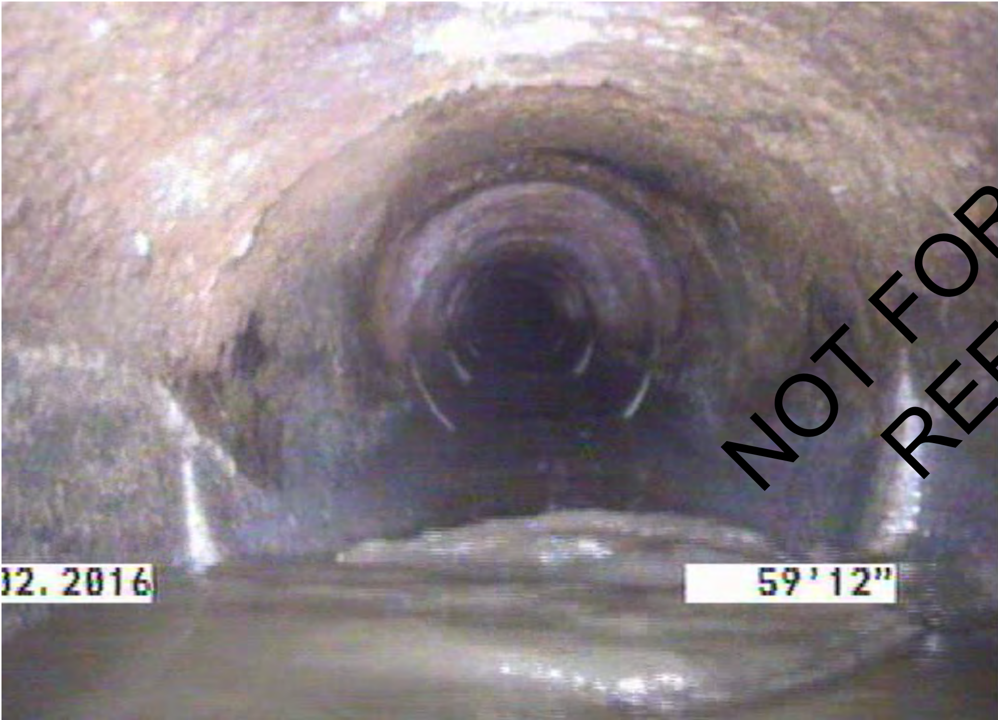
DEBRIS BETWEEN MH-NQL01M0134 & MH-NQL01M0135
