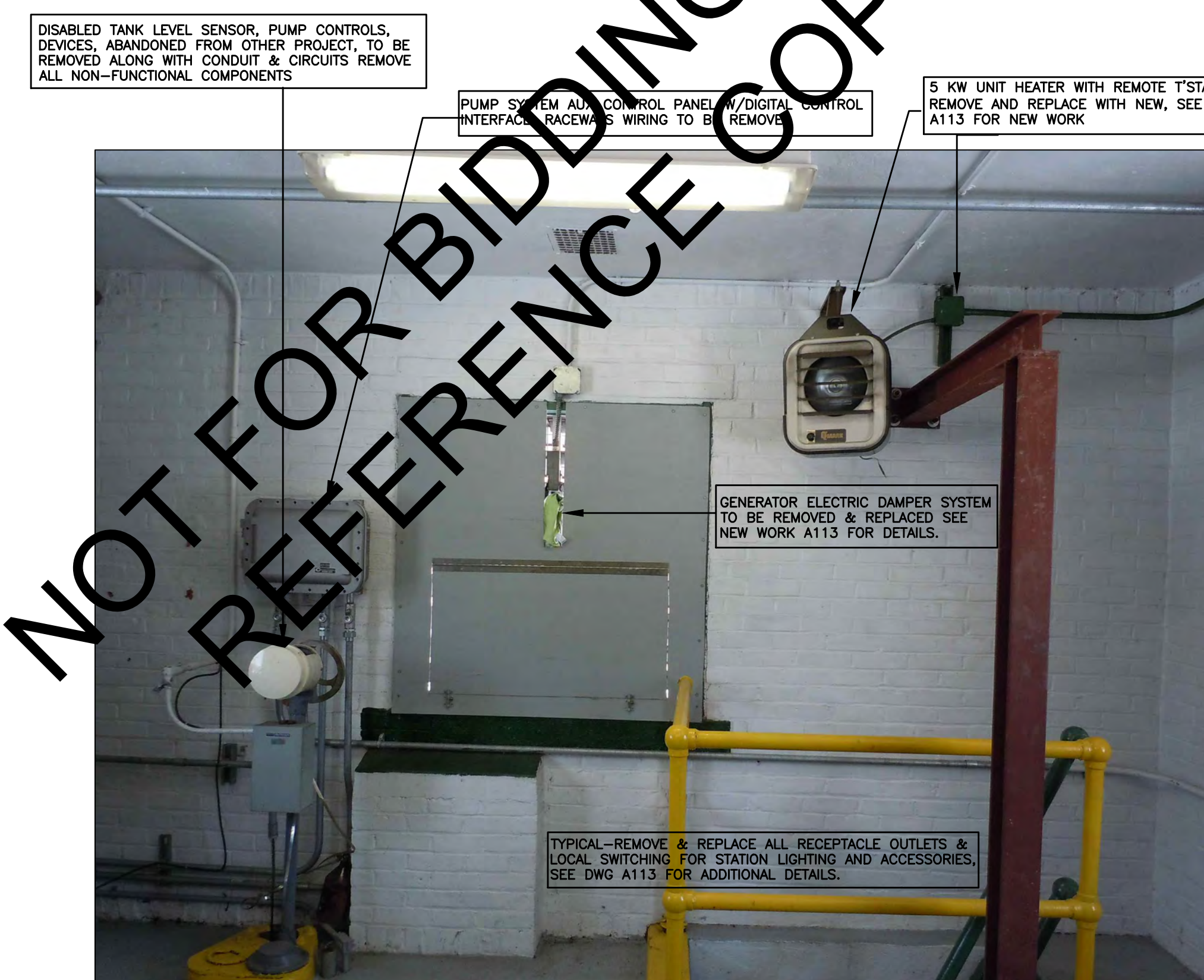
ELECTRICAL DEMO - NORTH ELEVATION
