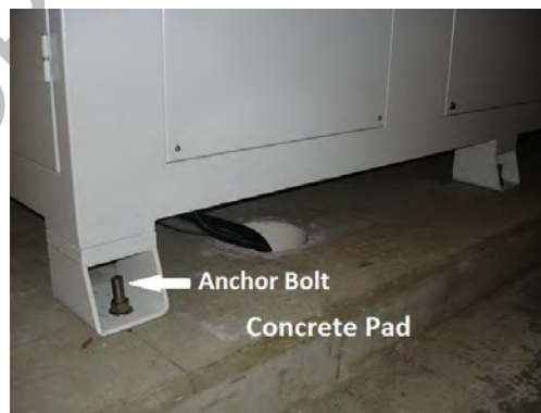
ANCHOR BOLT INSTALLATION
