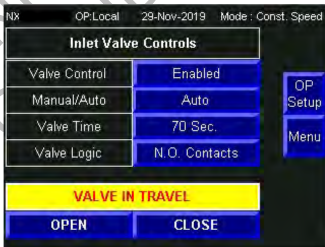
INLET VALVE CONTROL SCREEN
