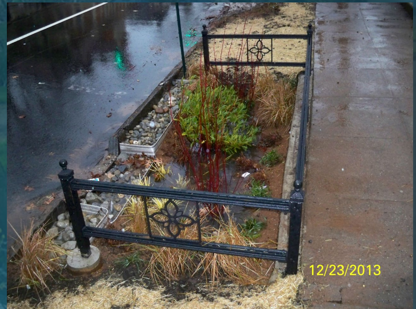
New Haven's First Bioswale Trumbull St near Whitney Av
